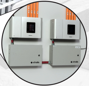
VESDA Early Warning Aspirating Smoke Detector
